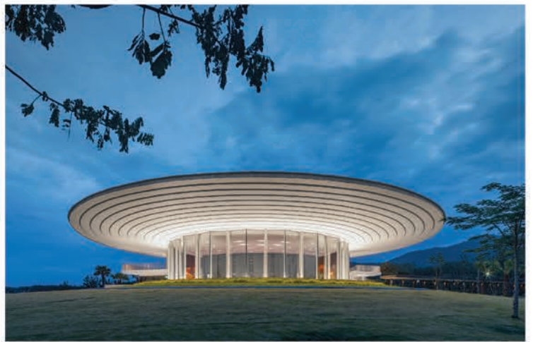
2015 VIDYASIRIMEDHI INSTITUTE OF SCIENCE AND TECHNOLOGY (VISTEC) Wang Chan Valley, Rayong
